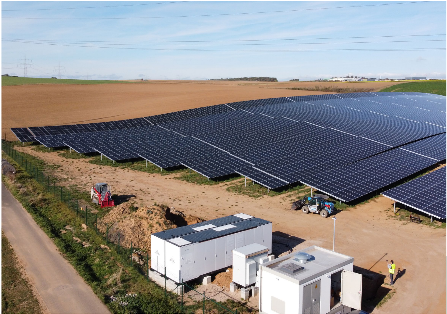
Solar plus Storage in Theilheim, Germany: A ground mounted system with one SG3125HV-30 inverter and two Sungrow PowerTitan ST2752UX storage systems
