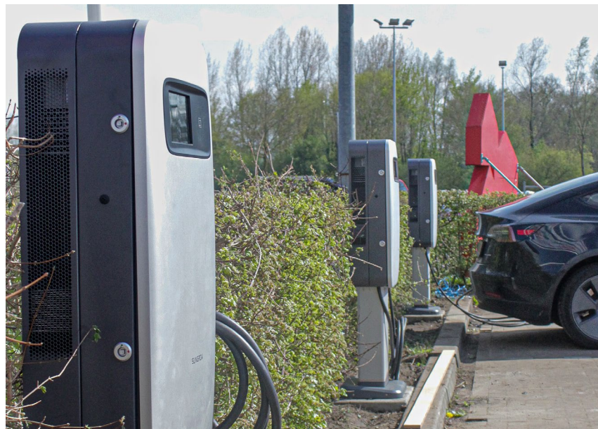
Fast Charging while shopping in Groningen, Netherlands: ten IDC30E pole-mounted DC Chargers
